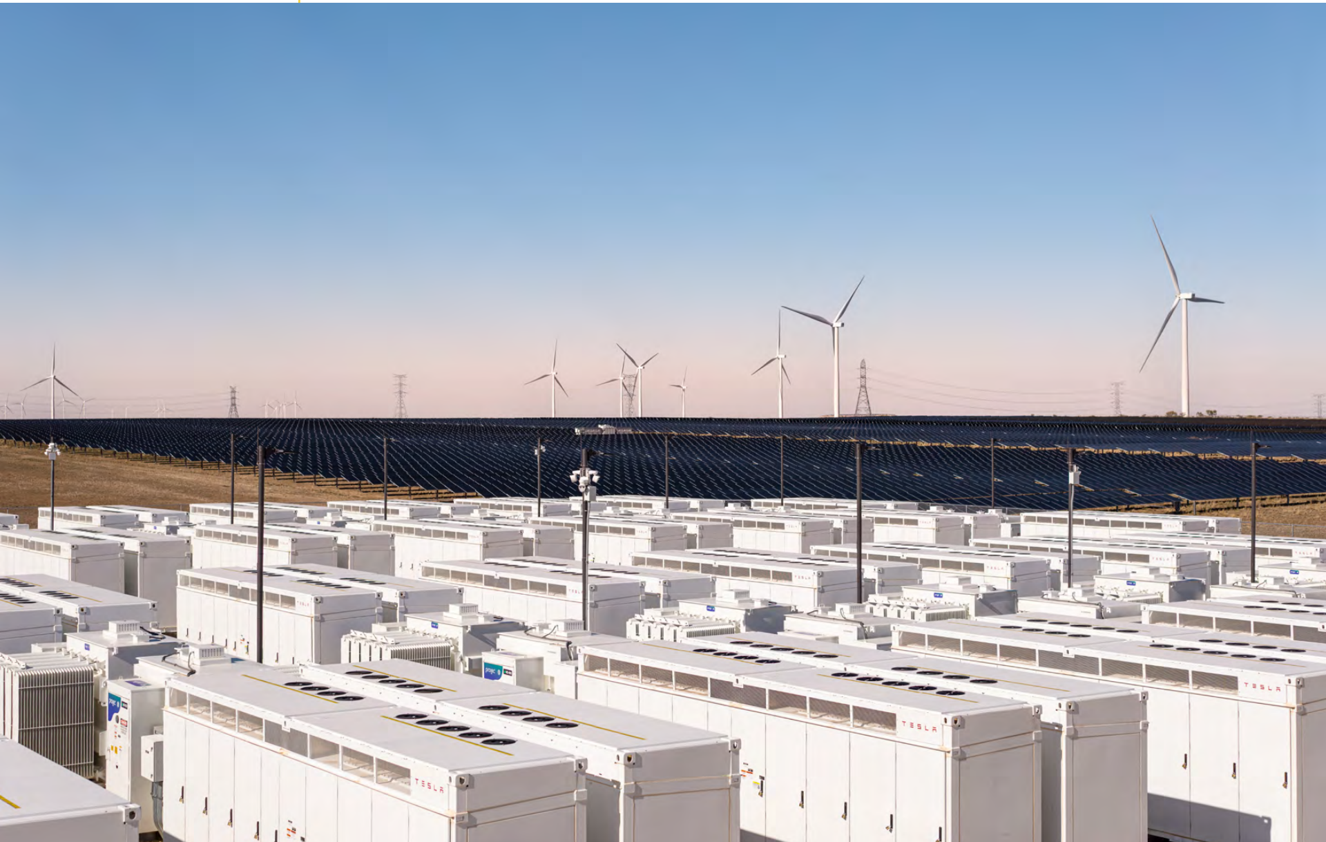
The Lumina Solar + Storage facility, located in Scurry County, Texas, generates 828 MWp of solar power and features 640 MWh of battery storage.
